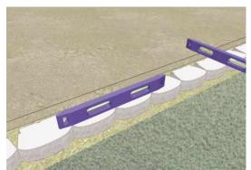
Step 2 - Install the First Course Set and level each unit of the base course front-toback, side-to-side across three-blocks. Align the base course units with a string line behind the tail of the blocks.
