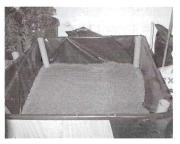
Bed fully constructed before soil is added. See the PVC pipes, the black plastic. Hydrocorals line the bottom and are then covered with felt and chicken wire.
